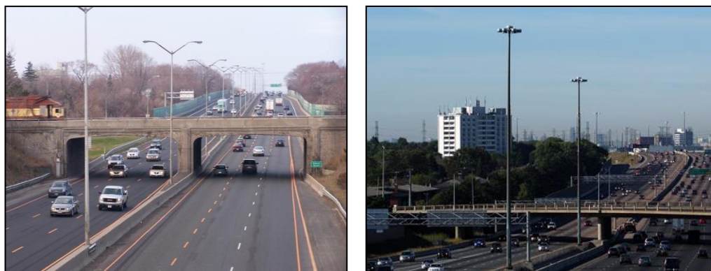
FIGURE 4-27: TYPICAL CONVENTIONAL (LEFT) AND HIGH MAST (RIGHT) ILLUMINATION
